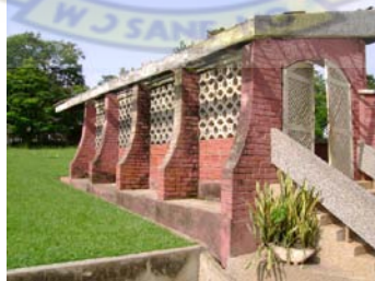
Fig. 2-13 Buttresses used as a feature on pavilion, library and fence wall (Source: Researcher's field survey)
