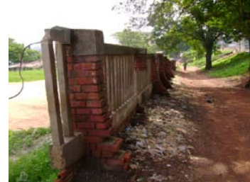
Fig. 2-13 Buttresses used as a feature on pavilion, library and fence wall (Source: Researcher's field survey)
