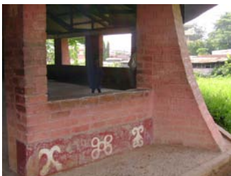
Fig. 2-13 Buttresses used as a feature on pavilion, library and fence wall (Source: Researcher's field survey)
