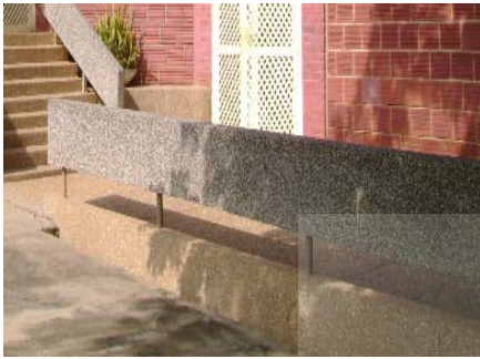
Fig. 2-14 Terrazzo finishing (Source: Researcher’s field survey)
