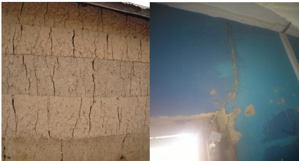
Plate 6: Series of Cracks in Buildings Resulting from Quarrying, Buoku and Papaasu
