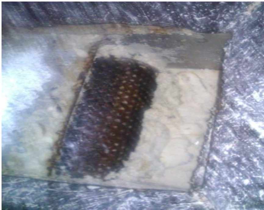
Figure A10: Grating surface rusting with time
