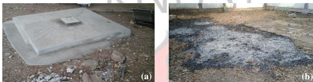
Figure 4.21: (a) Un-engineered pit for the disposal of pathological waste and (b) open air burning for the disposal of some non-hazardous waste.
