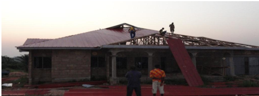
UNSAFE MATERIAL HANDLING 1
