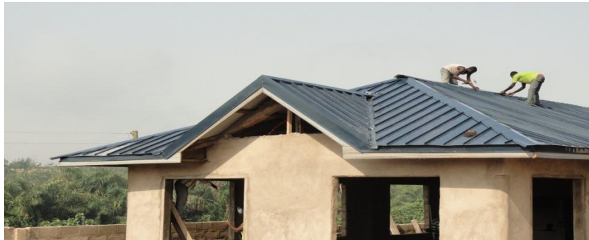
UNSAFE SHEET INSTALLATION 2
