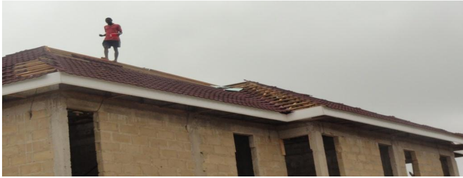
WRONG ACCESS ON ROOF 1
