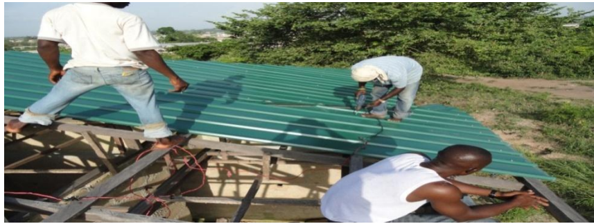
UNSAFE SHEET INSTALLATION 1
