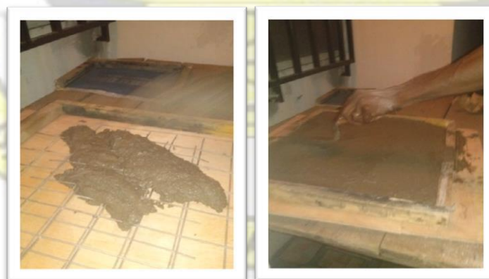
Plate 17: Preparing the mortar
