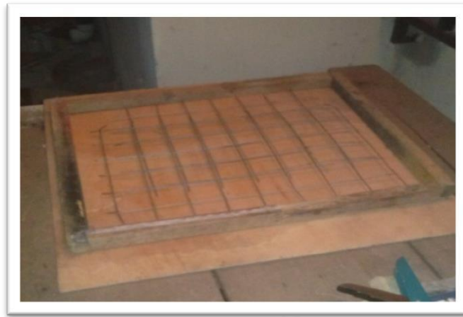
Plate 16: Prepared frame ready to receive the mortar
