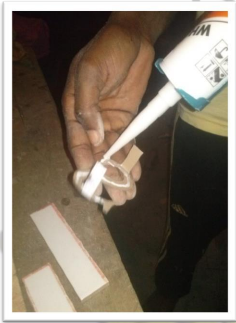
Plate 19: Applying silicone to back of font
