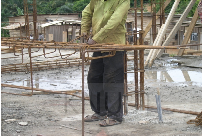
Steel benders working on reinforcement bars in foundation without gloves, helmets of safety boots
