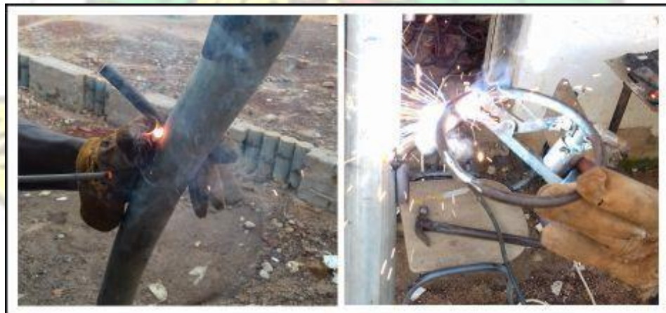
Plate 3.91: Welding the extensions to the pipe
