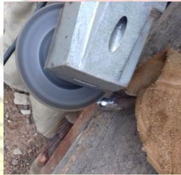
Plate 3.90: Grinding the extension
