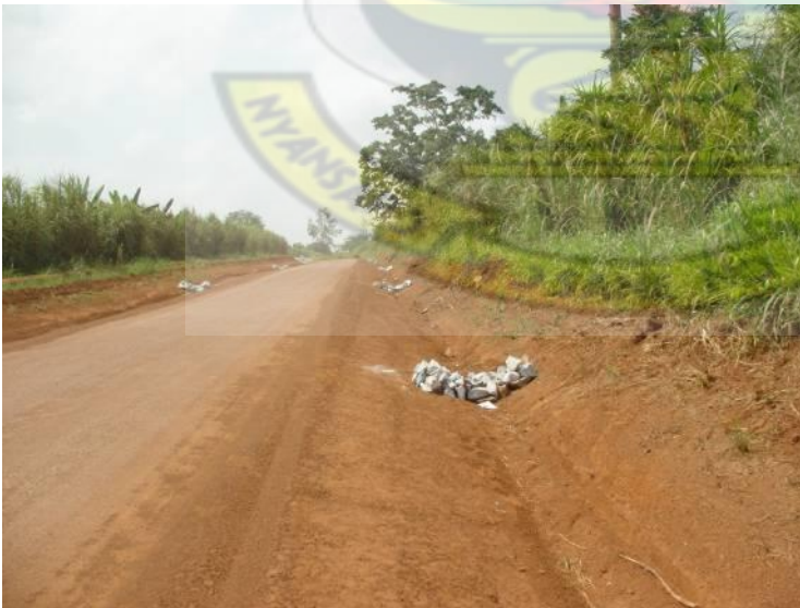
Figure 5. 14:- Newly Made Check Dams on Camp A – Ntoroso Road to Reduce Velocity of Runoffs and Aid Sedimentation.
