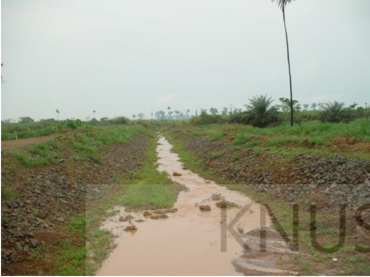
Figure 5. 13:- One of the Channels Created to Direct Runoffs from the Administration Area, Camp A and Plant Site to Sedimentation Basin ECD3
