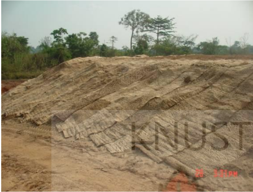
Figure 5. 15:- Covering Topsoil from the Subika Pit with Locally Made Jute Mat.
