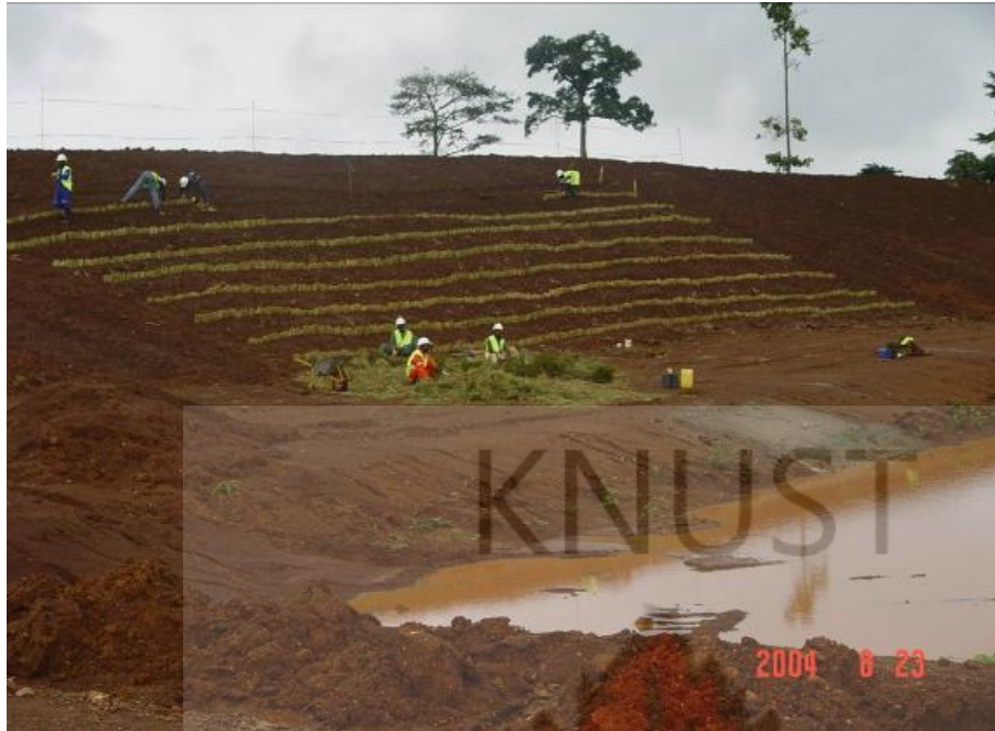
Figure 5. 16:- Newmont Workers Planting Grasses to Prevent Erosion Around a Sedimentation Dam
