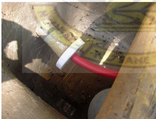
Plate 4. PVC pipe draining male urine into an 8 L container.
