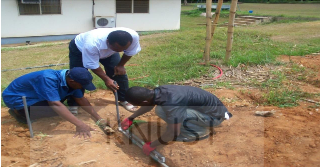
Figure 6. Pipe laying on the field in the various trenches
