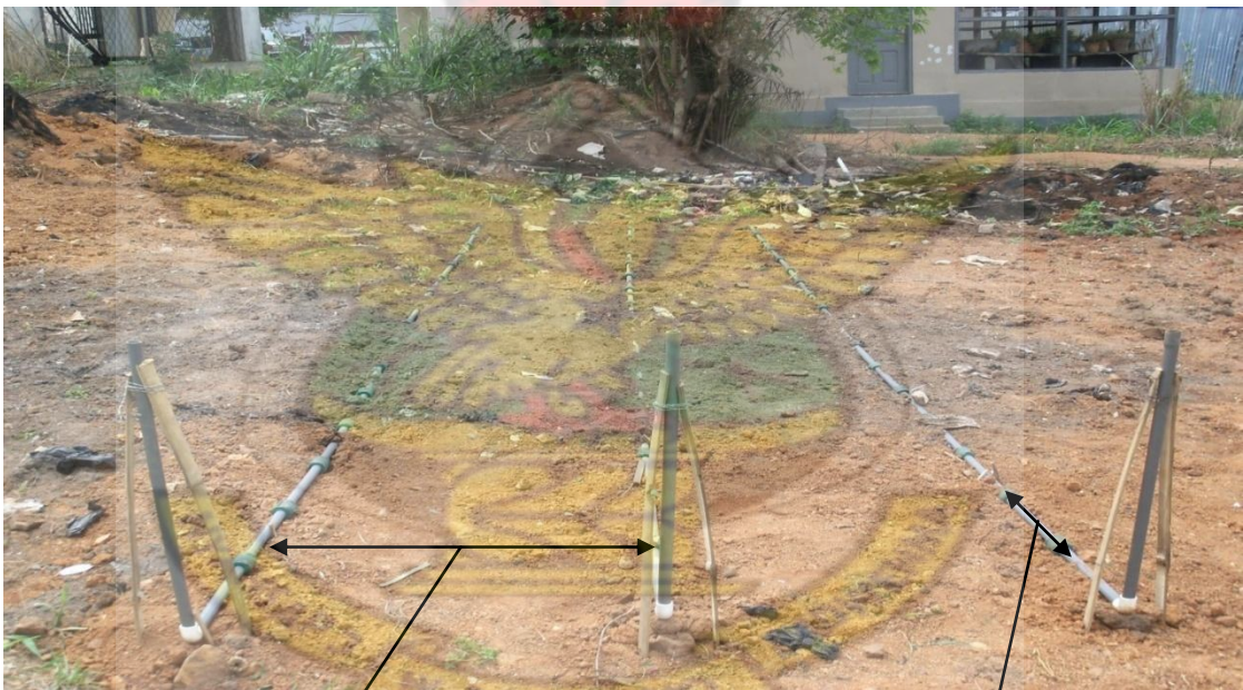
Figure 6. Pipe laying on the field in the various trenches
