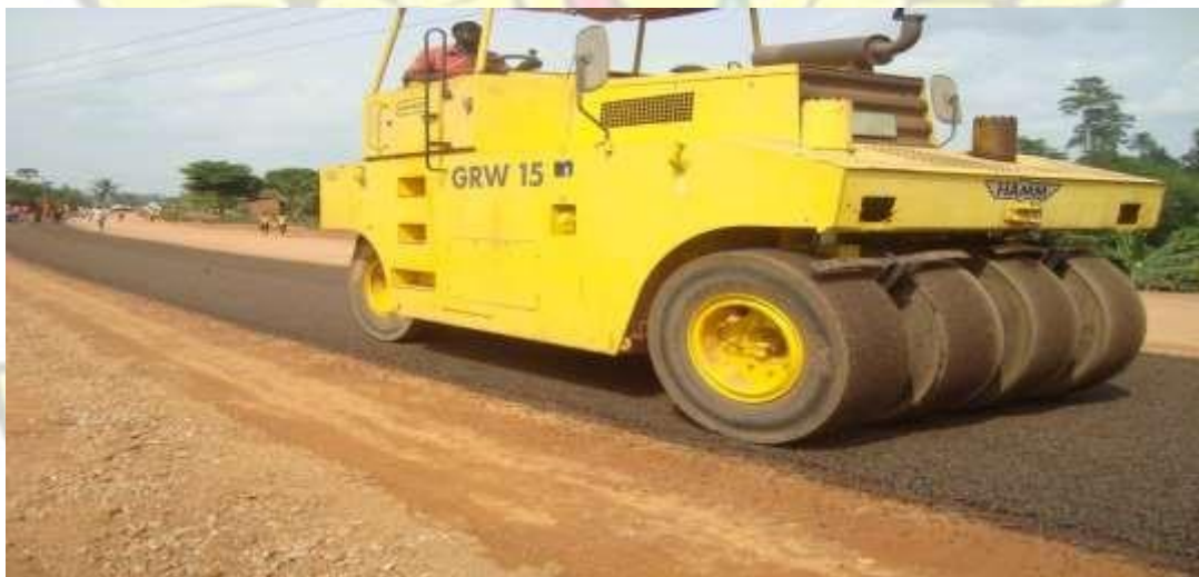
Figure 4.7. Rolling with pneumatic tyre roller
