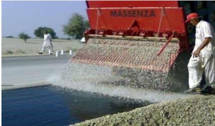
Figure 4.3. A typical electronic Chipping Spreader ( www.speedcraft.net/chippings-distributor )
