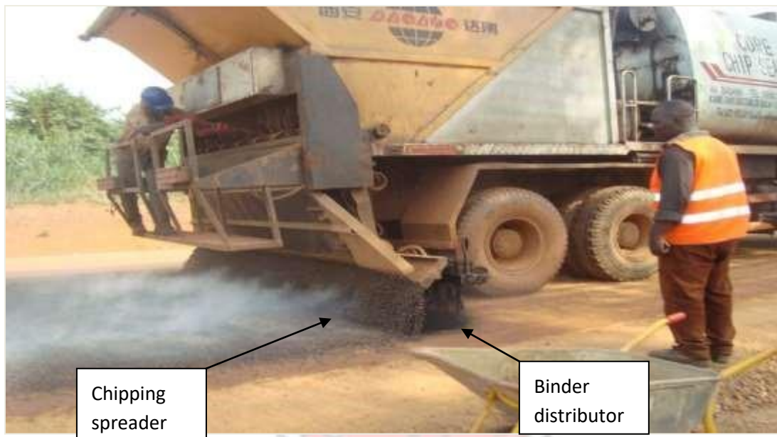
Figure 4.6. Electronic distributor and spreader
