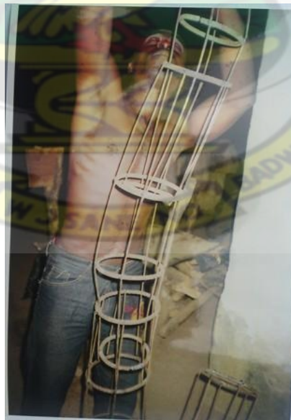
Figure 3.56 arranging the armature
