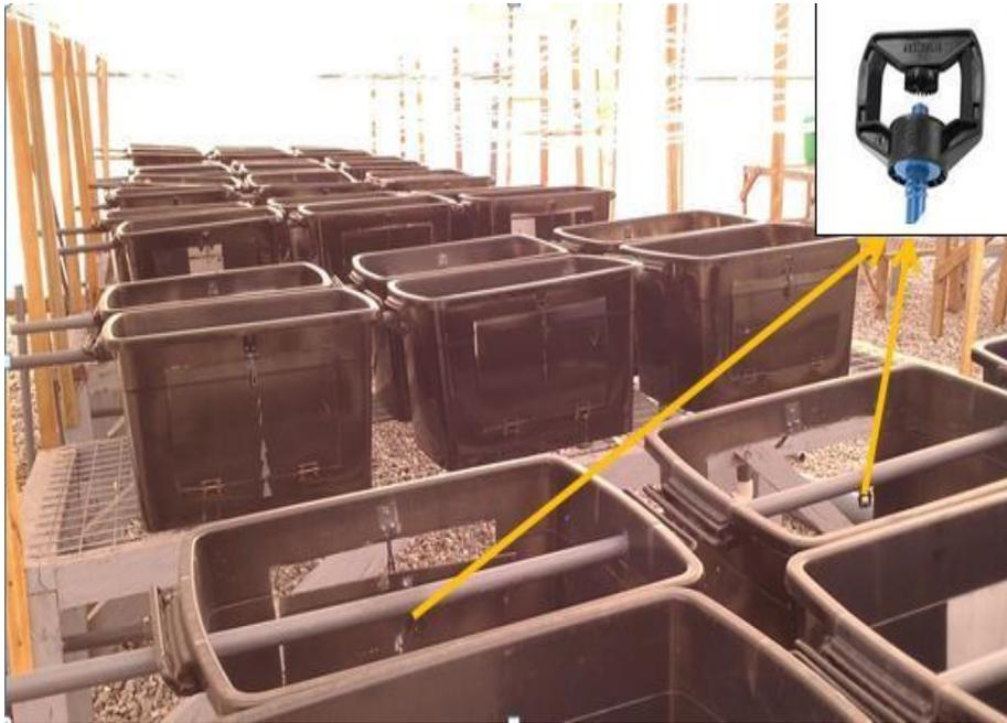
**Plate 3- 13 Feed Pipes showing misters**
