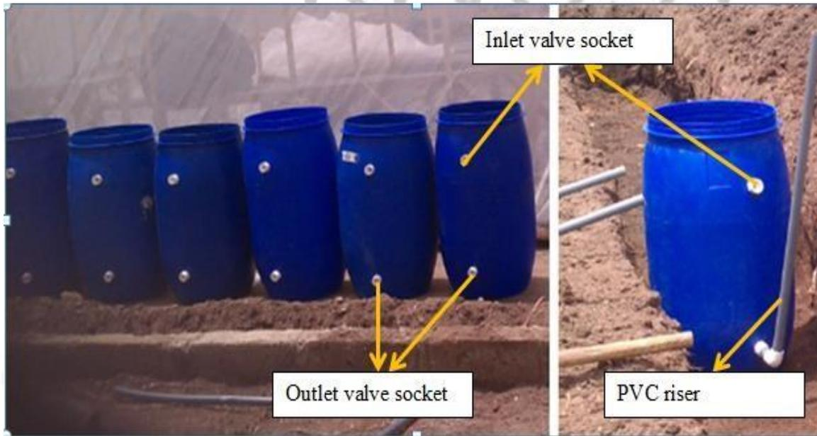
**Plate 3- 14 Feed tank showing inlet, outlet and riser**
