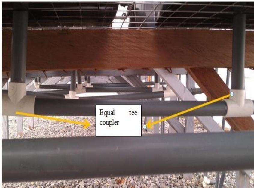
**Plate 3- 12 Setup showing drains with equal tee couplers**
