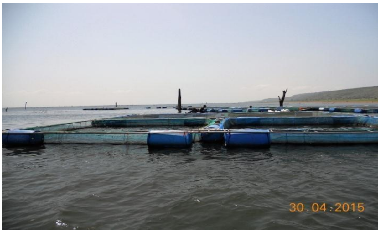
Figure 2.5: A square cage with galvanized pipe frames on the Lake Volta
