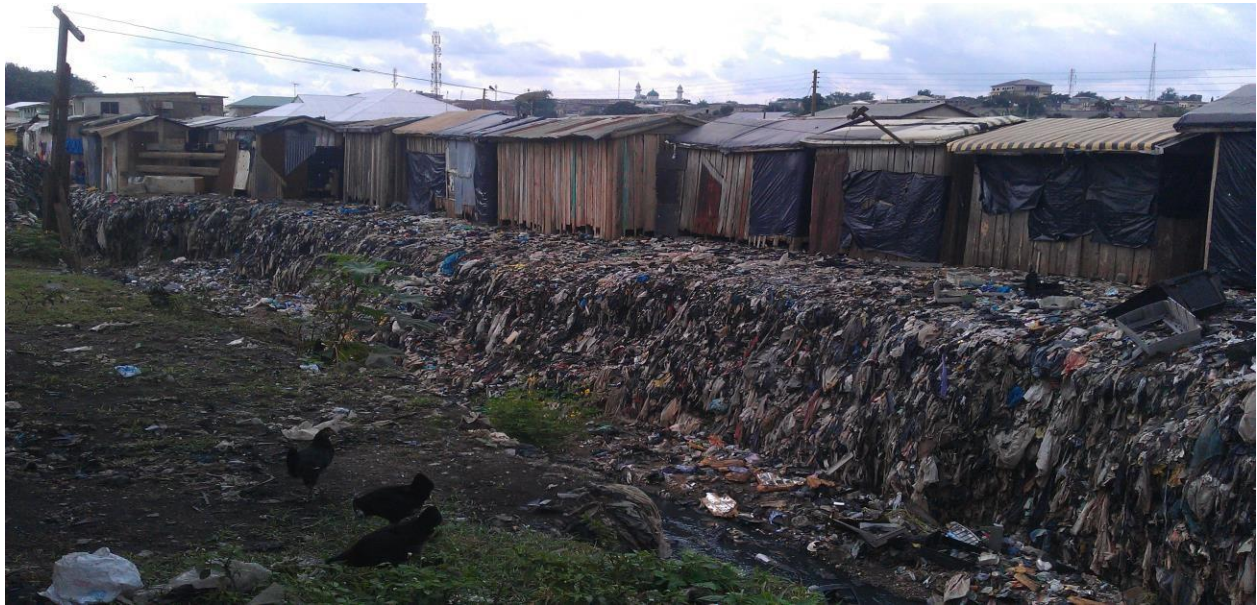
Figure 5.3: Drain choked with refuse connecting to the Aboabo River at Aboabo
