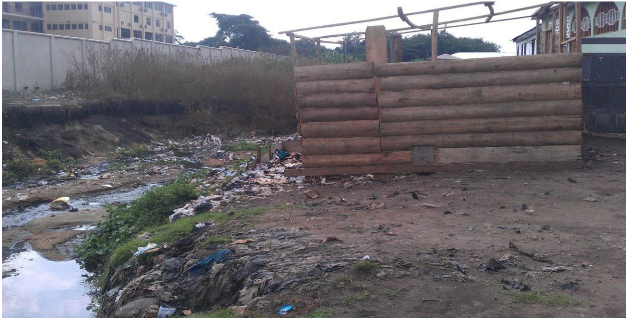
Figure 5.4: Poorly constructed drain within the Aboabo basin at Anloga
