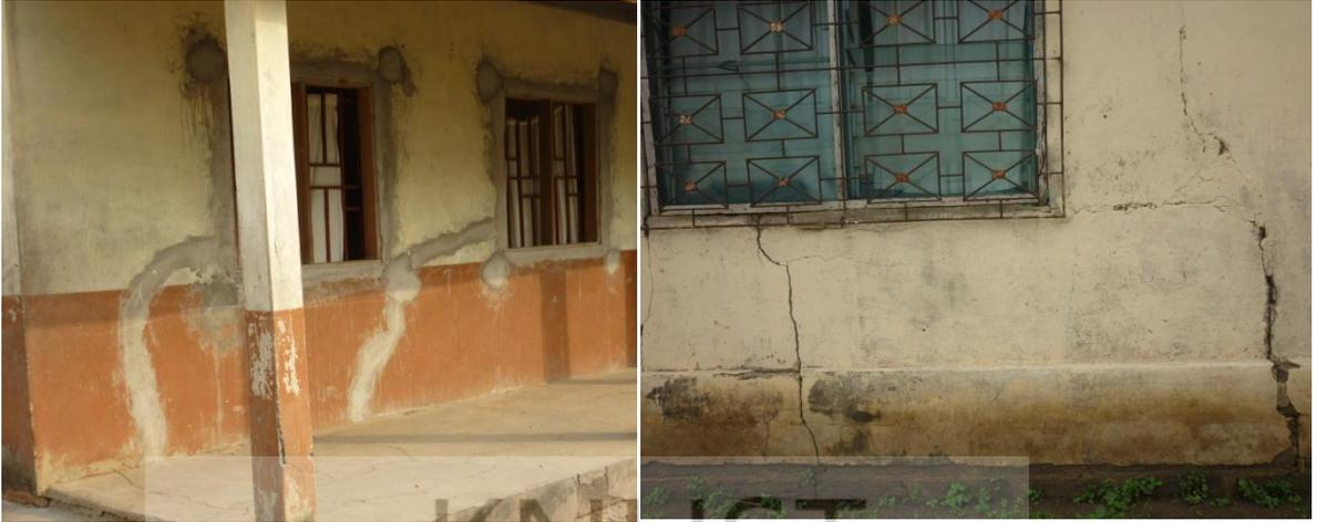
**Plate 1a. Deformation in building in the Accra Plains**
