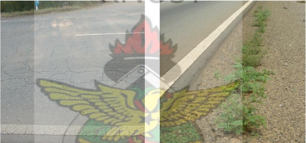
**Plate 1b. Cracking in pavement in the Accra Plains**
