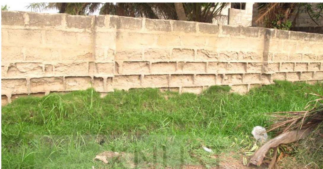
**Figure 5.10 Wall affected by flooding in Glefe.
