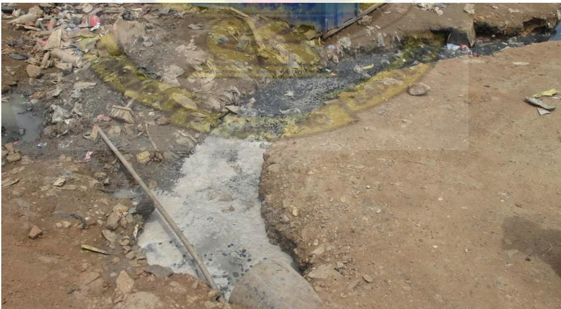
**Figure 5.28 Choked drain in Glefe.**
