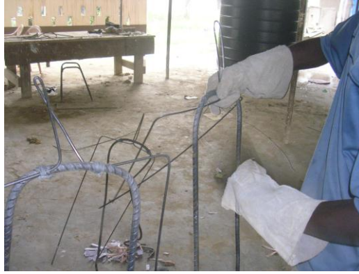
Plate lx Tying with binding wire
