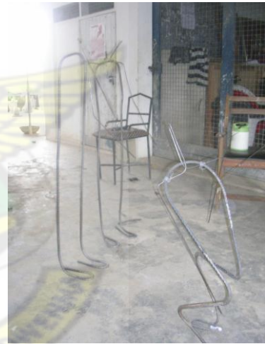
Plate lxii Assembling of constructed armature
