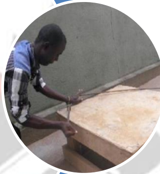
Bending of Iron Rods.
