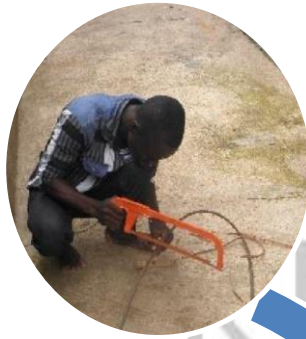
Cutting of Iron Rods to desired length
