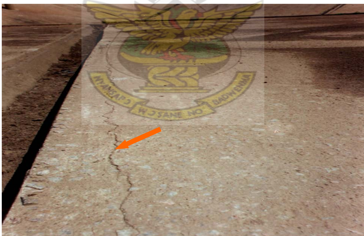
Figure 4.5 Cracks in the floor and the walls of storage reservoir at Nasia
