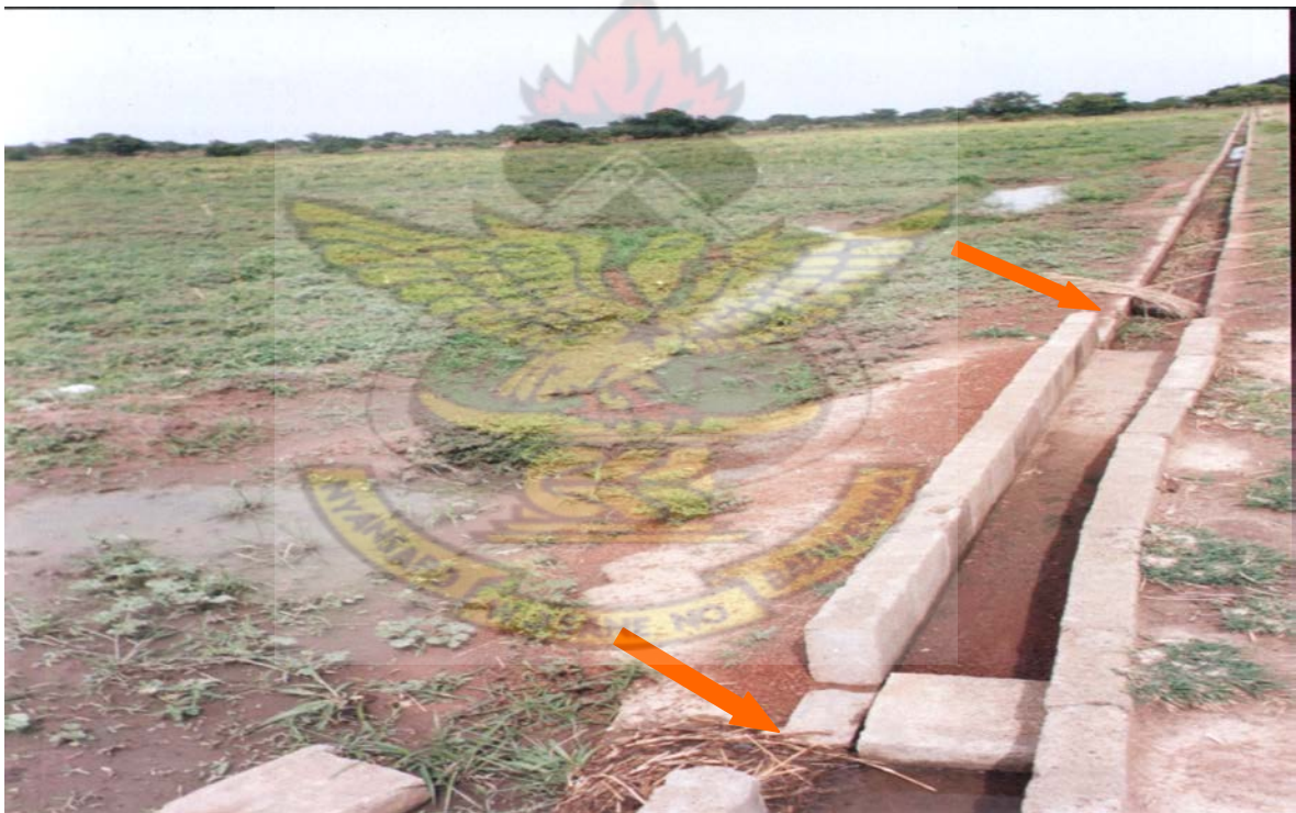
Figure 4.3 Broken canal at Nasia.
