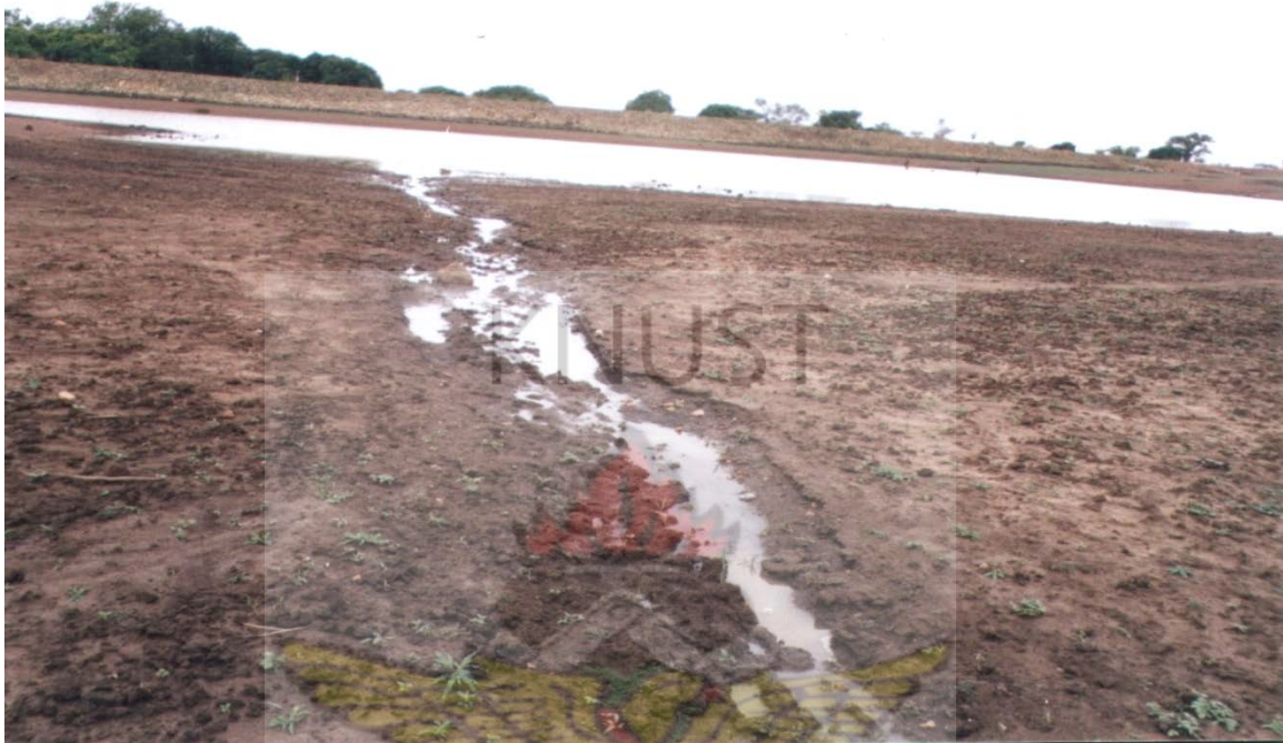
Figure 4.9 Silted Reservoir at Dorongo
