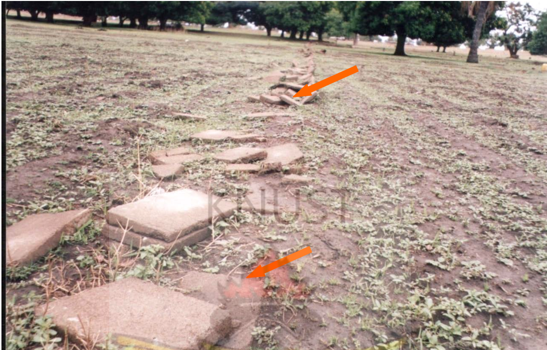
Figure 4.1: Poorly Constructed lateral at Dorongo
