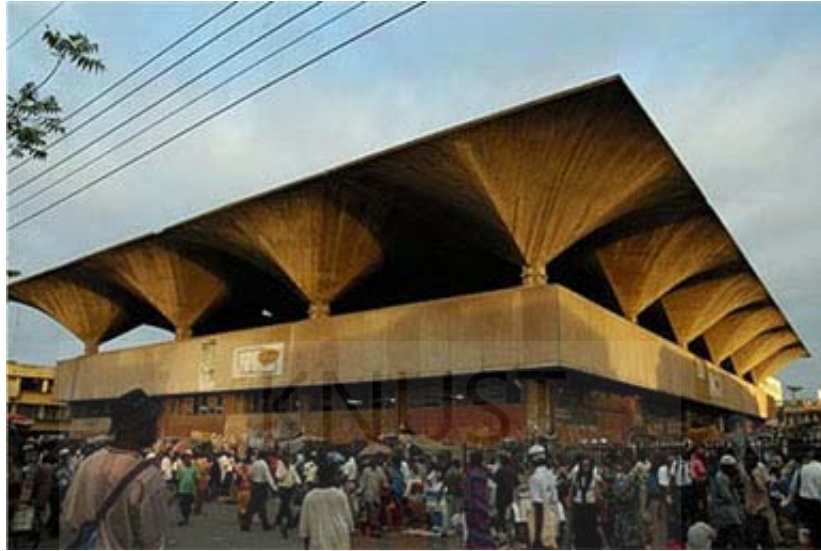
Fig. 4.23 Kariakoo market in Dar es Salaam showing its gigantic funnel-shaped roof to harvest rain.
