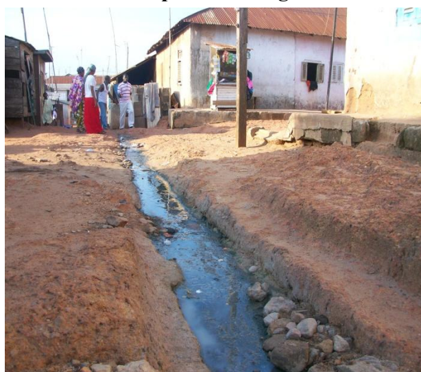
Plate 5.2. Open Drains at Kaase Causes Erosion and Expose Buildings' Foundation
