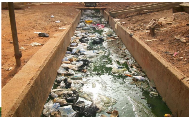
Plate A.1.1. Open Drains in Kumasi Filled with Solid Waste.
