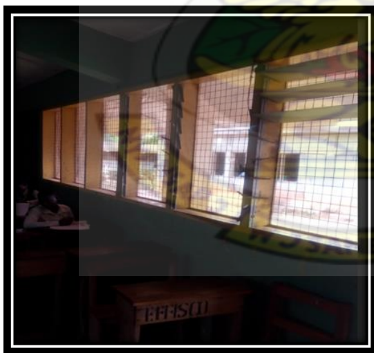
Plate 4.2: Classroom (broken louver blades)
