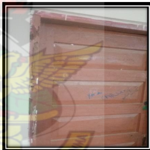
Plate 4.9: Decaying door frame
