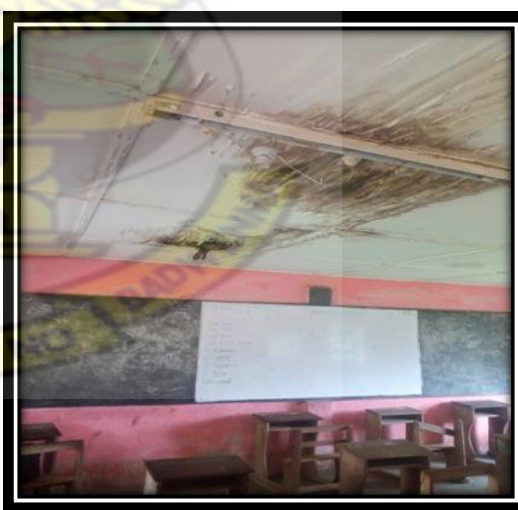
Plate 4.3: Classroom (leaking roof)
