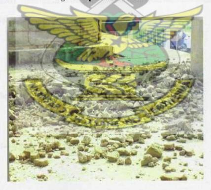
Fig 4.8 Crumbling blockwork on the site
