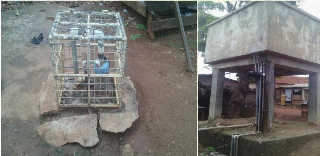
**Plate 4.4: Motorized Borehole with Storage**
