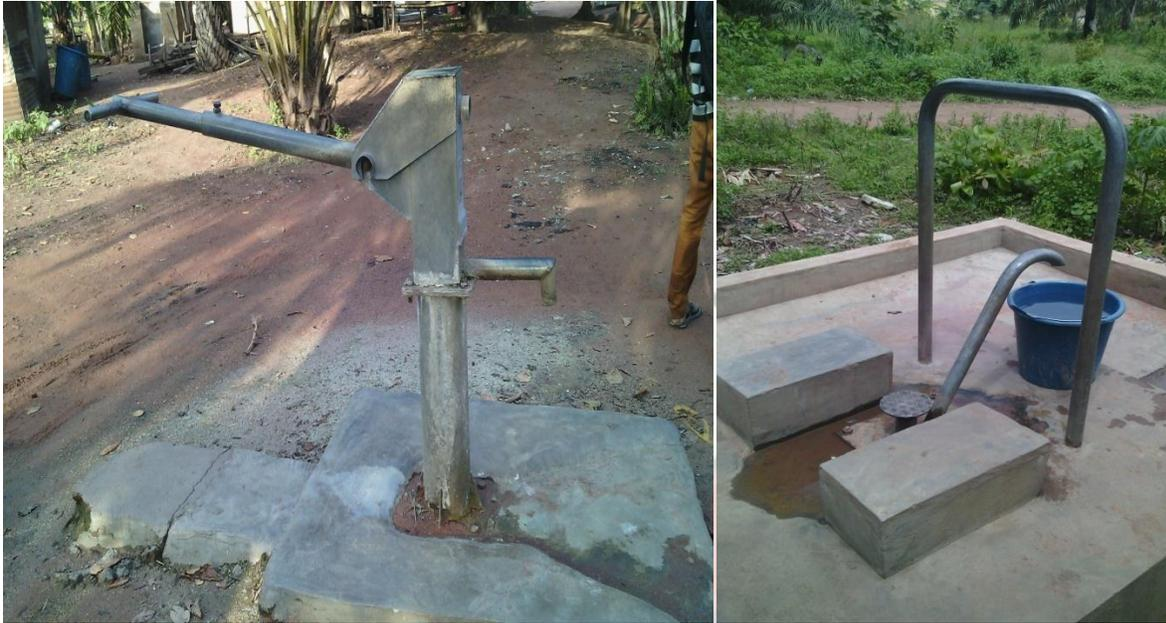
**Plate 4.3: Hand-Pump/Foot- Pump Boreholes**
