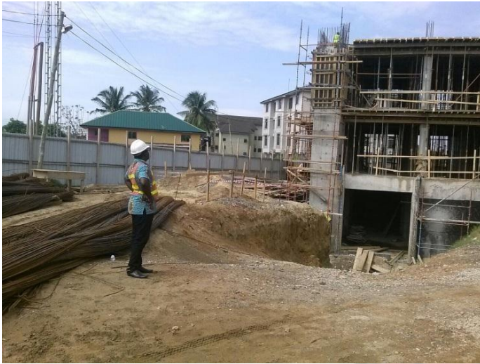
Plate 6: Steel members left in the open on the bare ground
