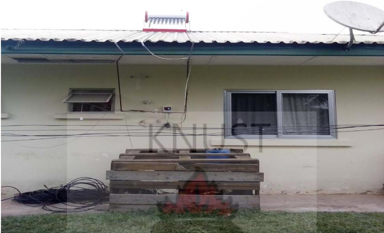
Figure 4.5 Picture of final installed SHW
