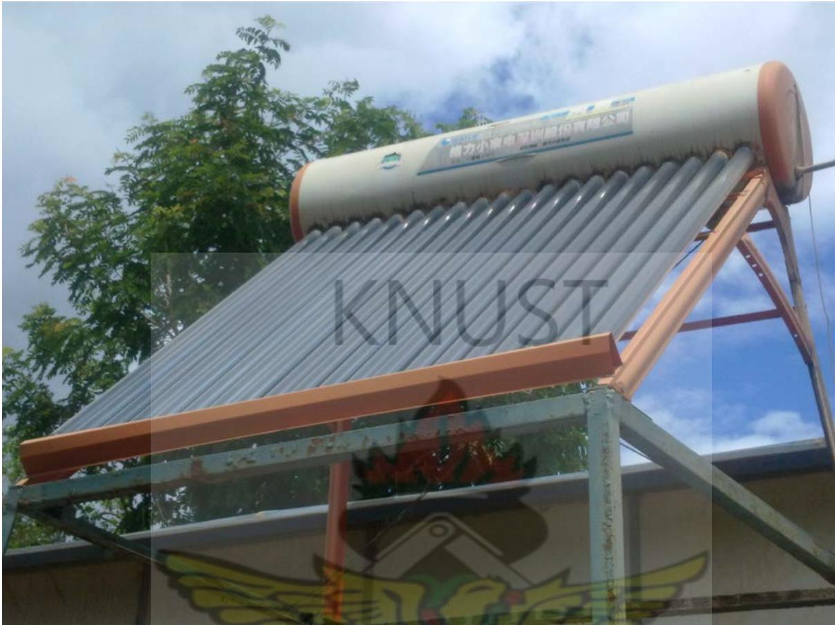
**Figure 2.7 an installed evacuated tube solar water heater at Bui, Ghana**
