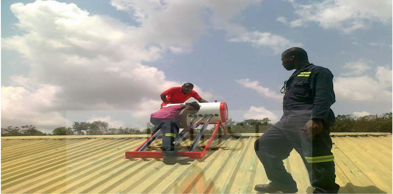
Figure 4.3b Plumbers installing evacuated tubes and pipes
