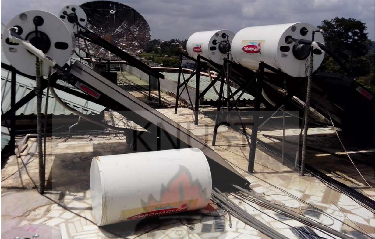
Figure 2.6 Flat plate collector water heaters installed at Anita Hotel in Kumasi, Ghana
