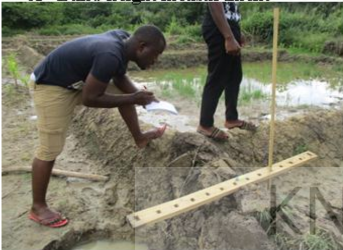
C - Construction of field channels to control water
