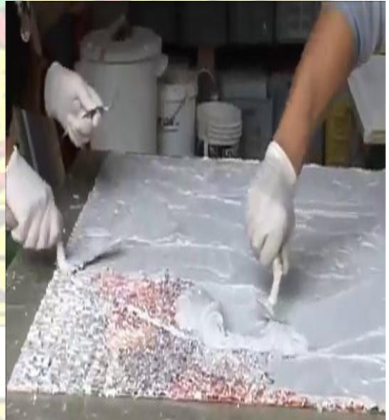
Figure 2.21b Mortar is applied to the back from
