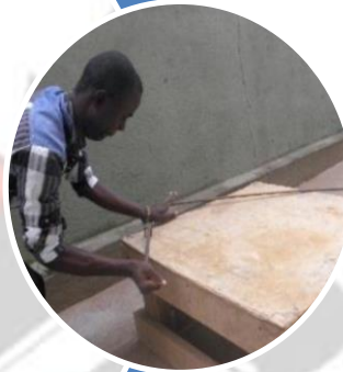
Bending of Iron Rods.
