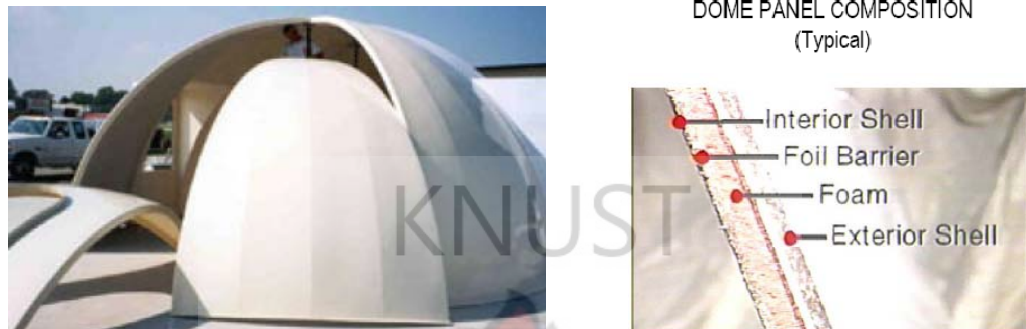
Figure 2.9: detail of fiberglass dome.
