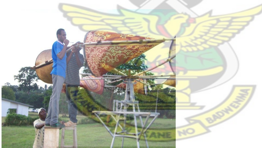
Figure 4.20 Mounting sails on rotor
