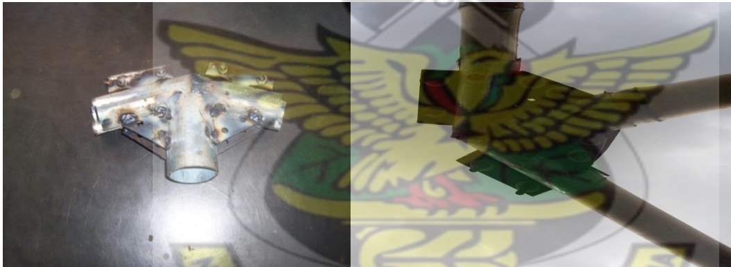
Figure 4.16 One end coupler & End coupler fitted with Bamboo
