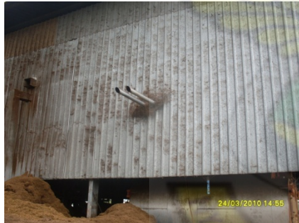
Plate 4.24 Corrugated galvanized steel cladding (Adansi Oil Mills)
