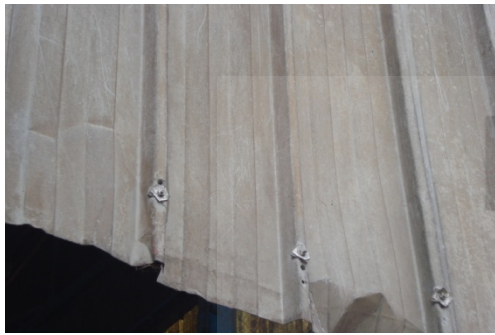
Plate 4.11 Corrugated aluminium cladding of the production block (Juabeng Oil Mills)
