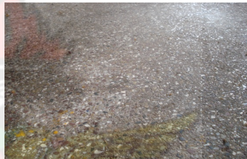
Plate 4.2 Terrazzo floor finish of the production block (Juabeng Oil Mills) (Source: author's field survey)
