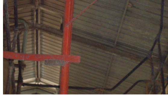
Plate 4.23 Horizontal member of portal frame (Adansi Oil Mills) (Source: author's field survey)
