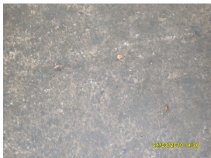
Plate 4.18 Monolithic concrete screed
