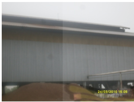
Plate 4.25 Roof form allowing for smoke ventilation (Adansi Oil Mills)
